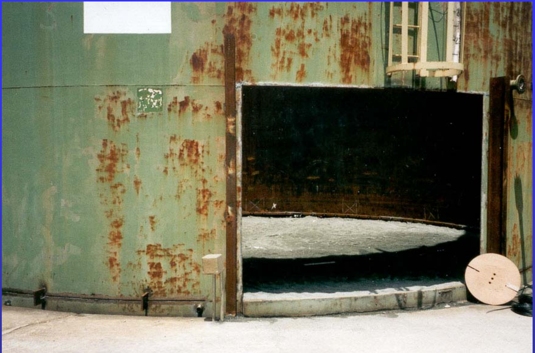
New Floor Installation on Existing AST
