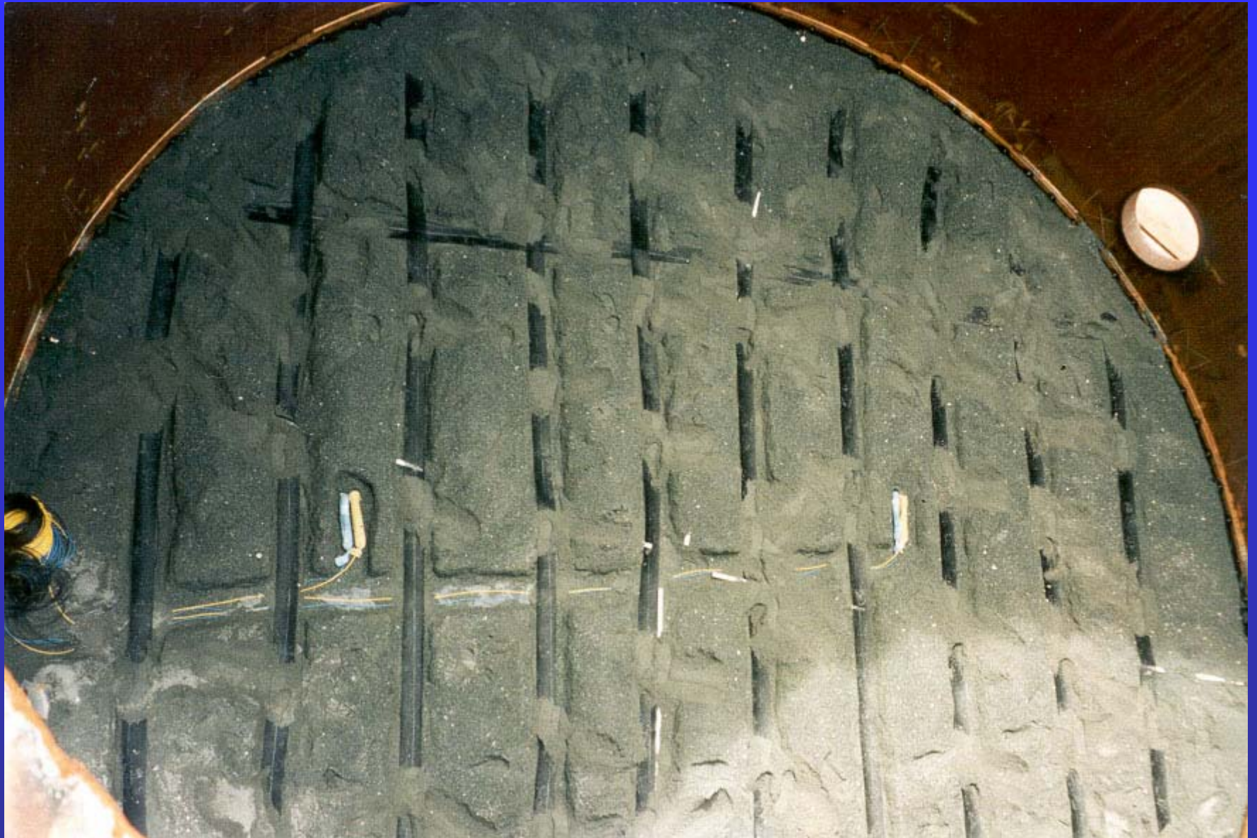
CP Installation on Rebottomed Tank
