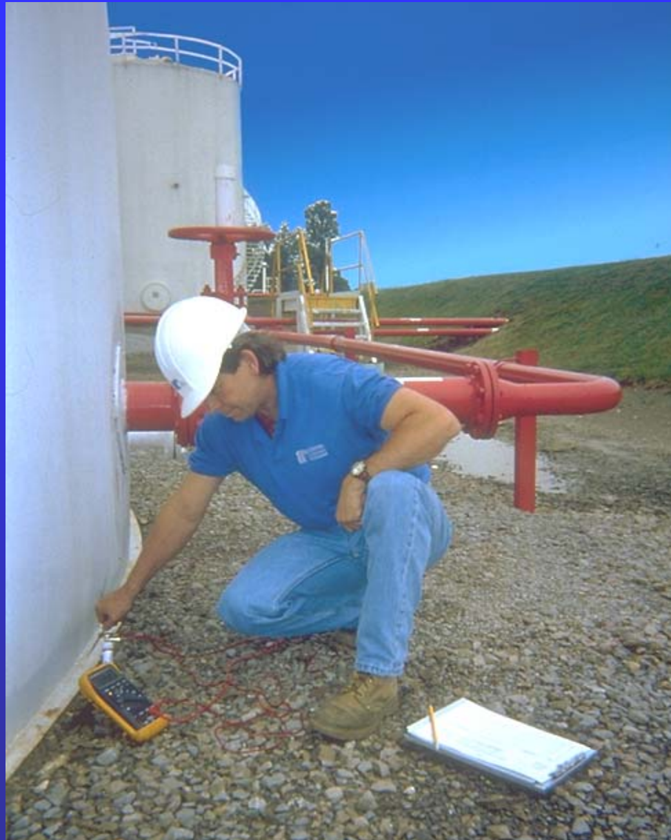
Cathodic Protection Monitoring
