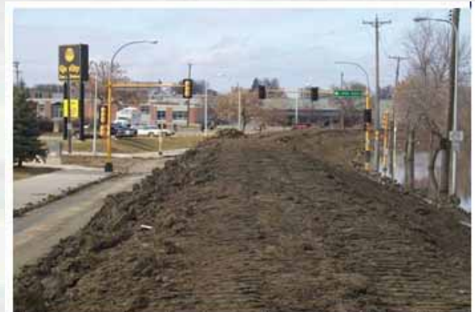
An Emergency Levee Protects the City at Second Street during the 2001 flood.
