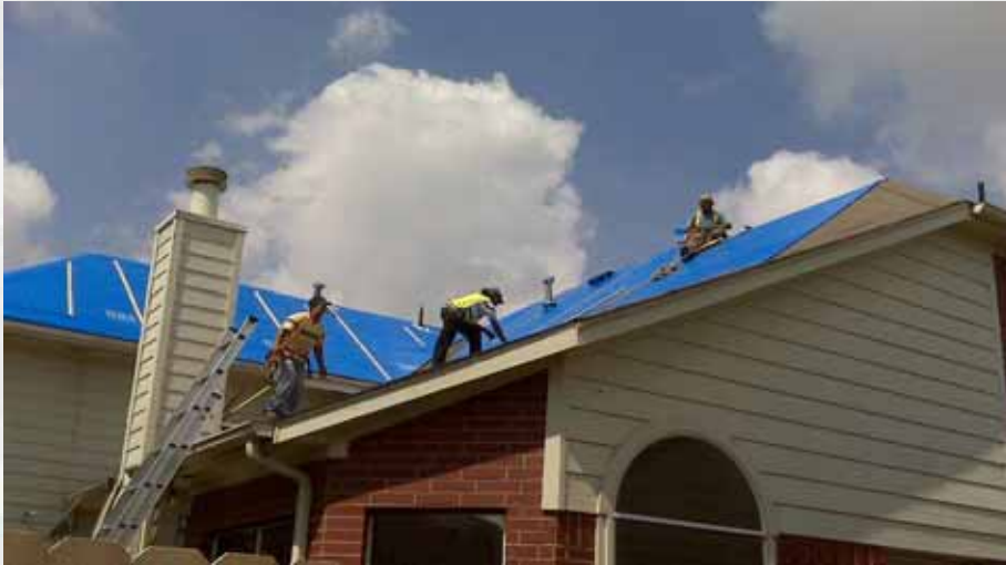
Temporary Roofing
